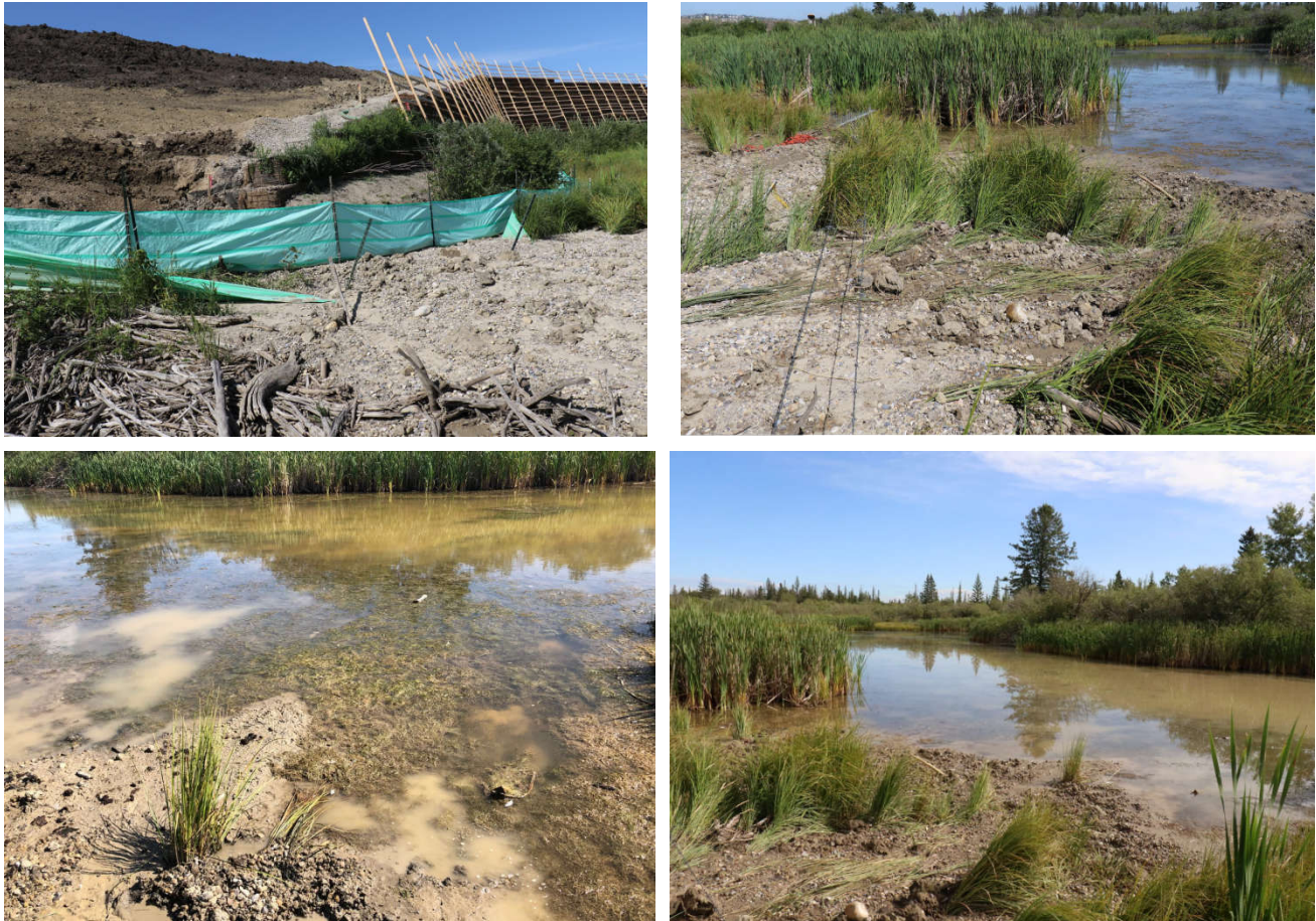
Figure 28: 19 th August 2019. Spill from construction site into Beaver Pond (note: spill occurred sometime before 19 th – new sediment fence has been erected); bottom right photo taken 5 days later shows additional sediment has washed into wetland following very heavy rain on 22 nd August
