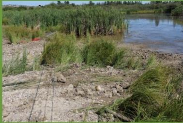
Sediment mitigation failure with coarse infill slide into the Beaver Pond, August 2019
