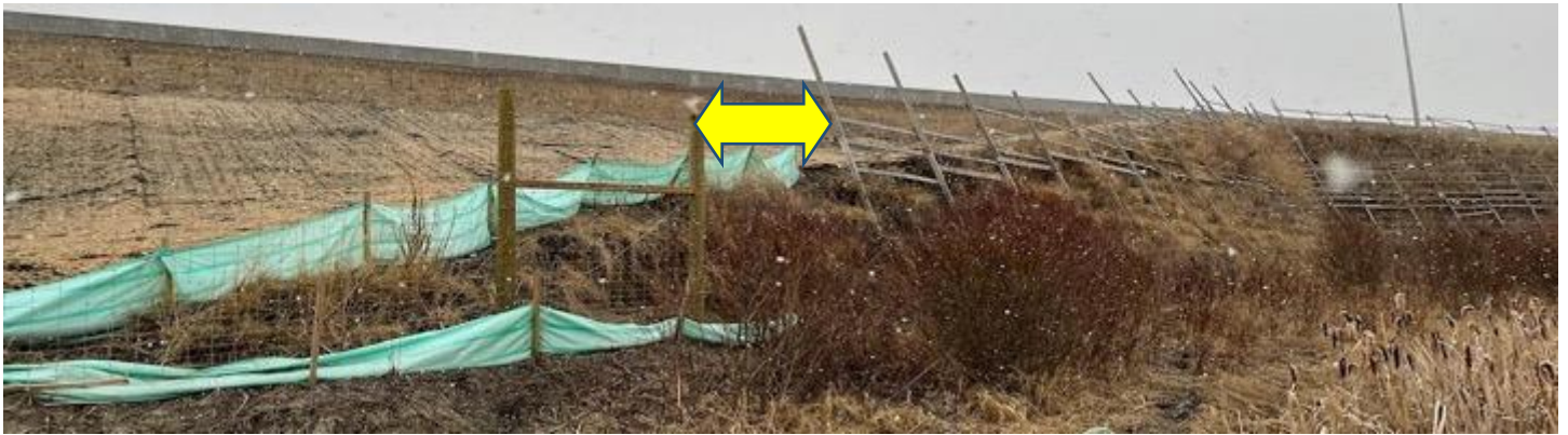
Figure 17. A visible gap at the fencing end exits at the start of the retaining wall, highlighted by the yellow arrow, was first observed in early 2022 west of the Beaver Pond and south of the retaining wall. Green fencing in the photo is erosion control fencing.
