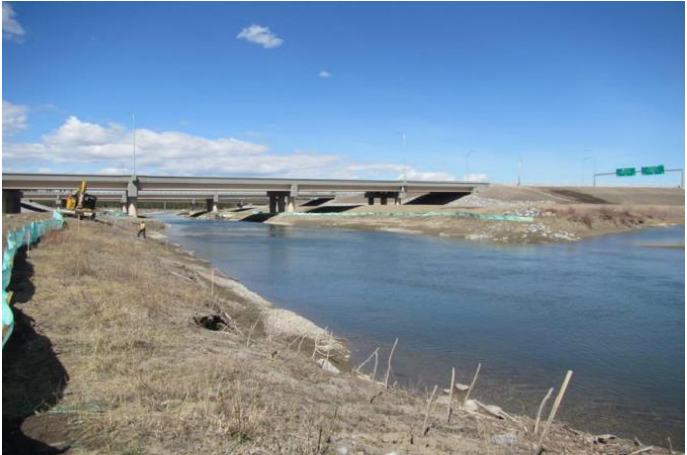
Figure 14. View looking Northwest, from the south bank of the Elbow River over the SWCRR showing the wildlife corridors in May 2021. Workers can be seen on the south bank using heavy equipment along the realignment corridor for willow staking. (Photo taken by Golder during the May 2021 Monthly Wildlife Monitoring Report 6 ). Green fencing visible on both sides of the river is erosion control fencing and is not a part of temporary or permanent wildlife fencing.
