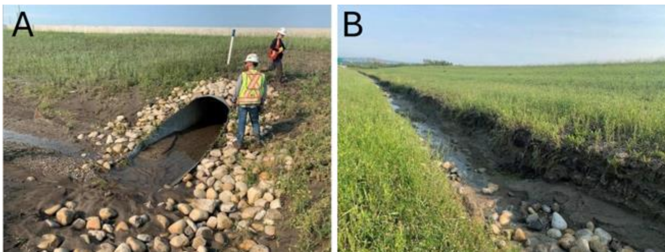
Figure 34A and B Silt inundation of western culvert berm (A) and channel erosion within ditch alignment (B) after rain event. (Taken From Hemmera WAIR 65 )
