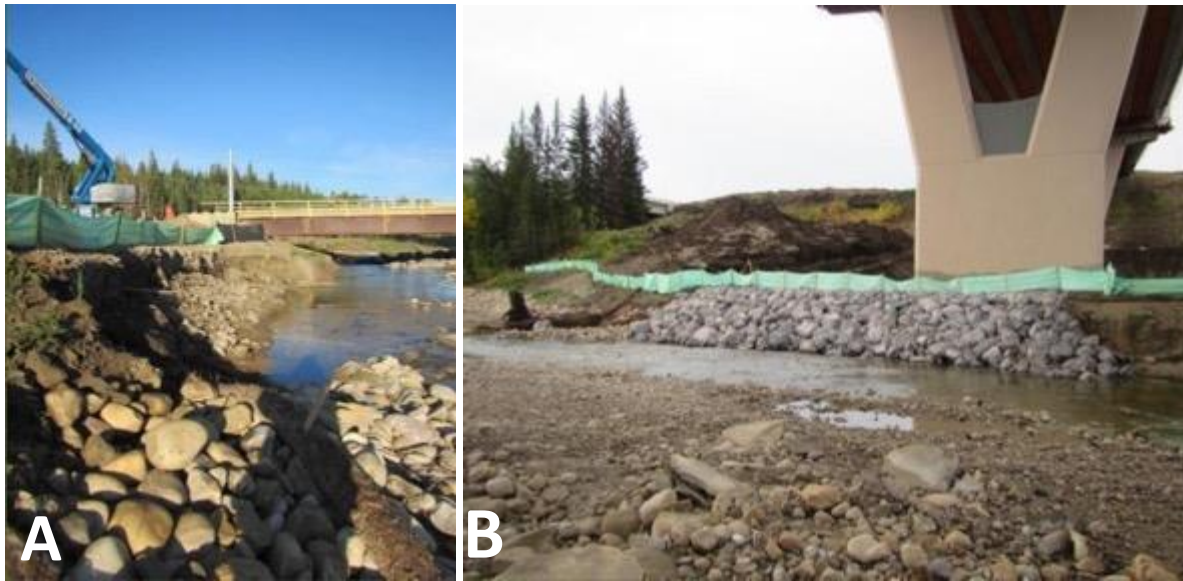
Figure 39A and B. Photo A is taken facing westward showing the erosion on the southern back of Fish Creek, under and east of the local bridge. (Photo from KGL August 2019 Monthly Wildlife Monitoring Report 6 ). Photo B is taken facing southeast under the bridge showing repaired erosion south of Fish Creek diversion. (Photo from KGL September 2019 Monthly Wildlife Monitoring Report 6 ).
