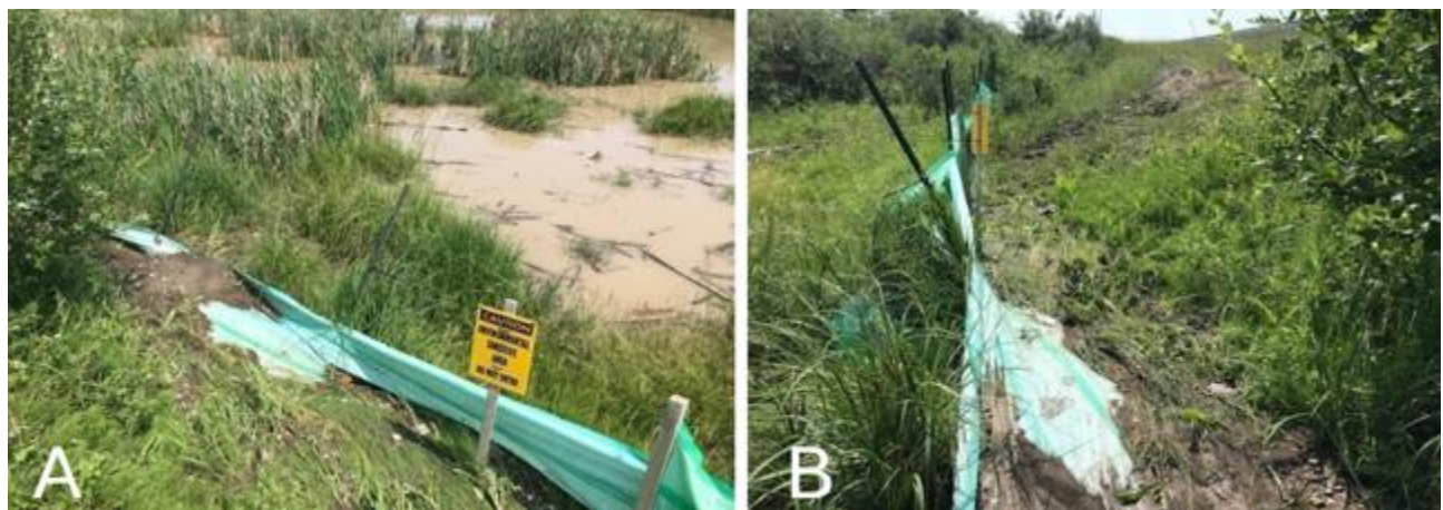
Figures 36A and B. Photographs of the Beaver Pond in the Weaselhead, identified as ‘Environmental Sensitive Area’, following sediment and course infill mitigation failure resulting in contamination of the wetland. Note the same failed mitigation measure used on top of the buried sediment fencing. (Taken July 3, 2021)
