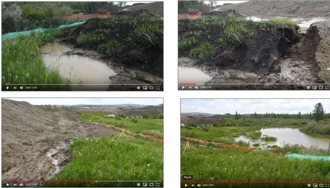
Figure 26: Still images from video captured on 23 rd June 2018; by Jeff Brookman available online 12 showing sediment flowing from the construction site (left) into Beaver Pond (right)
