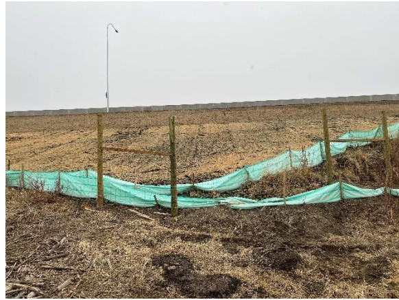
Figure 33. Hemmera WAIR photo 12 shows the installation of the erosion control matting in the summer of 2021. The following image was taken April 19, 2022 of the erosion control matting and fencing.
