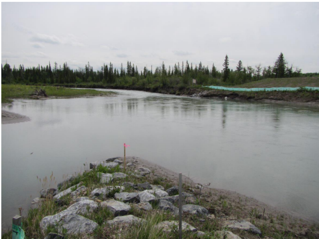
Figure 40. View facing east from the north bank of the river showing water levels at the Elbow River realignment and temporary fencing on the south side of the river. Photo taken by Golder during the June 2021 track survey.
