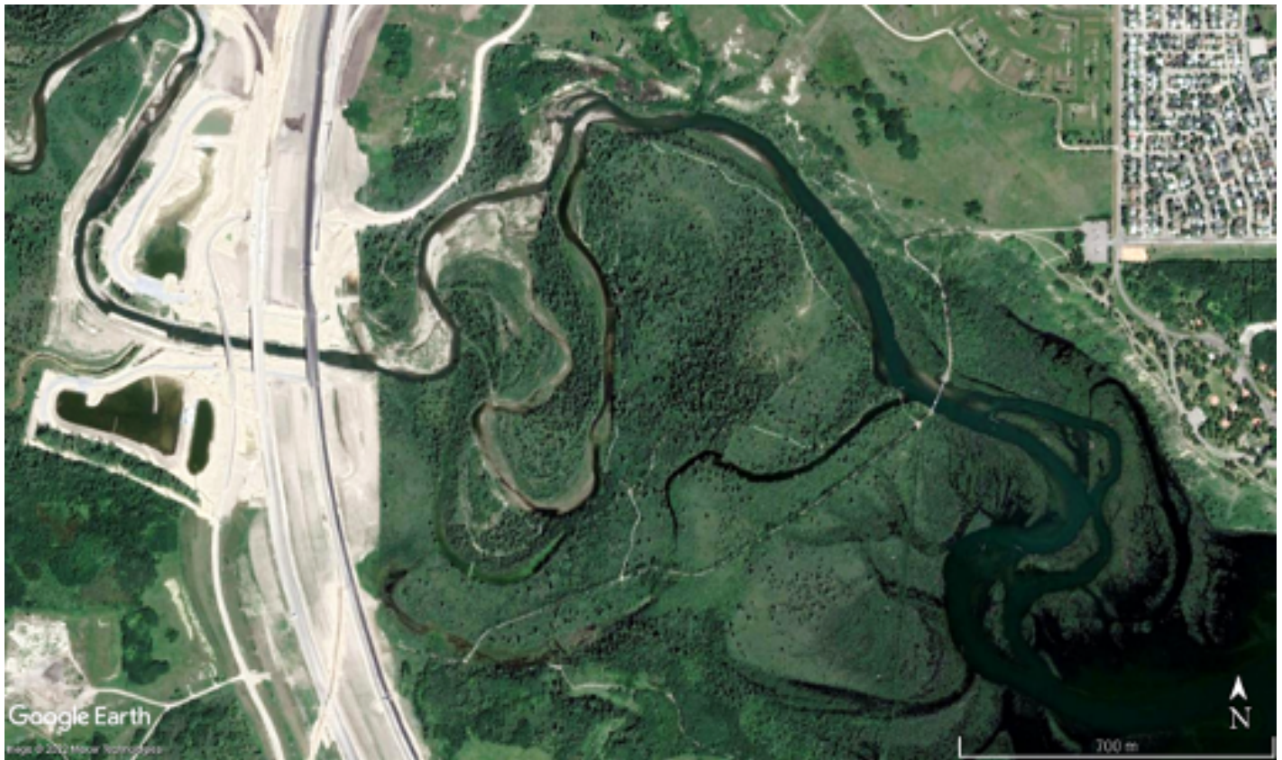
Figure 3. An aerial view of the Weaselhead with the SWCRR under construction and the different hydrological features indicated (Aug. 4, 2020).
