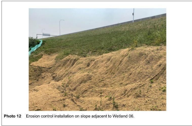
Figure 33. Hemmera WAIR photo 12 shows the installation of the erosion control matting in the summer of 2021. The following image was taken April 19, 2022 of the erosion control matting and fencing.
