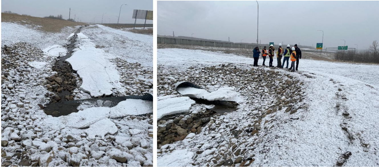
Figure 35. April 19, 2022, visit to inspect drainage and stabilization improvements.
